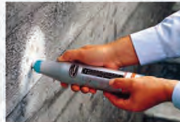
Testing with Rebound Hammer
